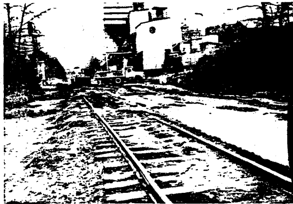
Fouled ballast at Bird's Mill Milepost 478.6
