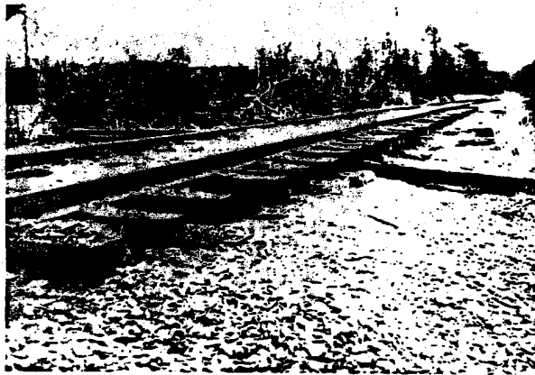
Item 8, Track Inspection Report 065: Insufficient ballast (washout) at Milepost 477.2
