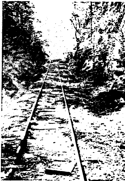
Rocks and slide in drainage ditch Milepost 455.6
