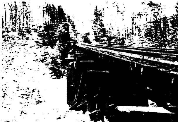
Bridge 458.4: Showing irregular surface on deck plate girder span
