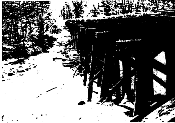
Item 6, Track Inspection Report 064, showing driftwood against piling Bridge 462.3
