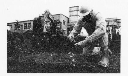
USPCI carefully removes contaminated soil around a Texas Eastern Pipeline Company compressor station near Shermans Dale, Pennsylvania – while the station remains in service. Tainted earth from this and several more sites along the pipeline is disposed of at USPCI's Grassy Mountain facility in Utah.
