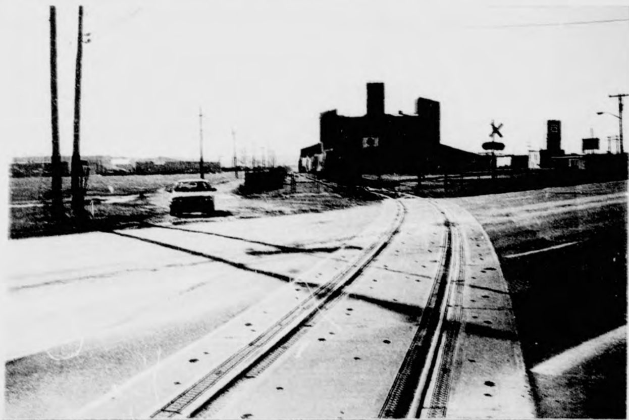
Photo I - View at Kentucky Street grade crossing. Note that crossing is not protected by crossing gates and that the flashing lights are not on cantilevers. Crossing would have to be upgraded if railroad traffic is to increase.
