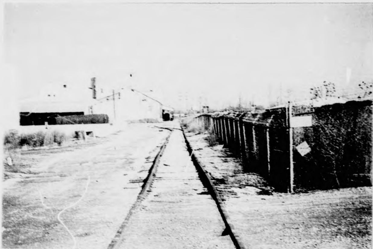
Photo I - View at Kentucky Street grade crossing. Note that crossing is not protected by crossing gates and that the flashing lights are not on cantilevers. Crossing would have to be upgraded if railroad traffic is to increase.
