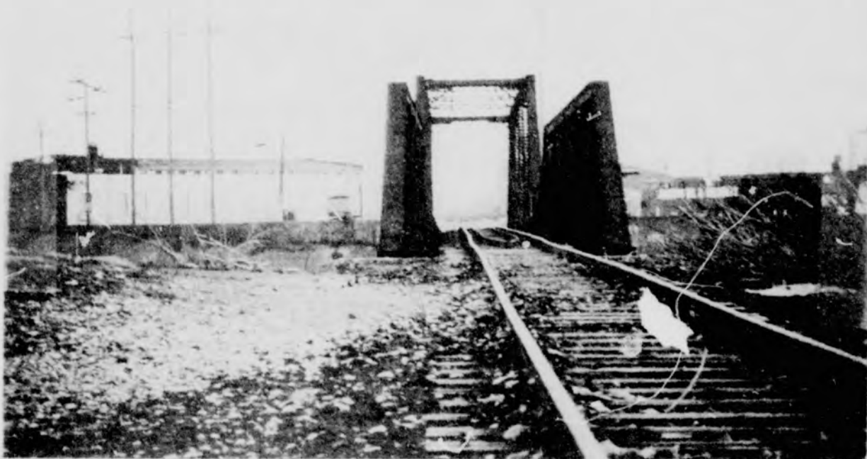
Photo K - View of bridge over Eagle Creek on Conrail track. Note severe dip in track at and off bridge - also some light construction of through truss span. Whole truss span is deteriorated severely.
