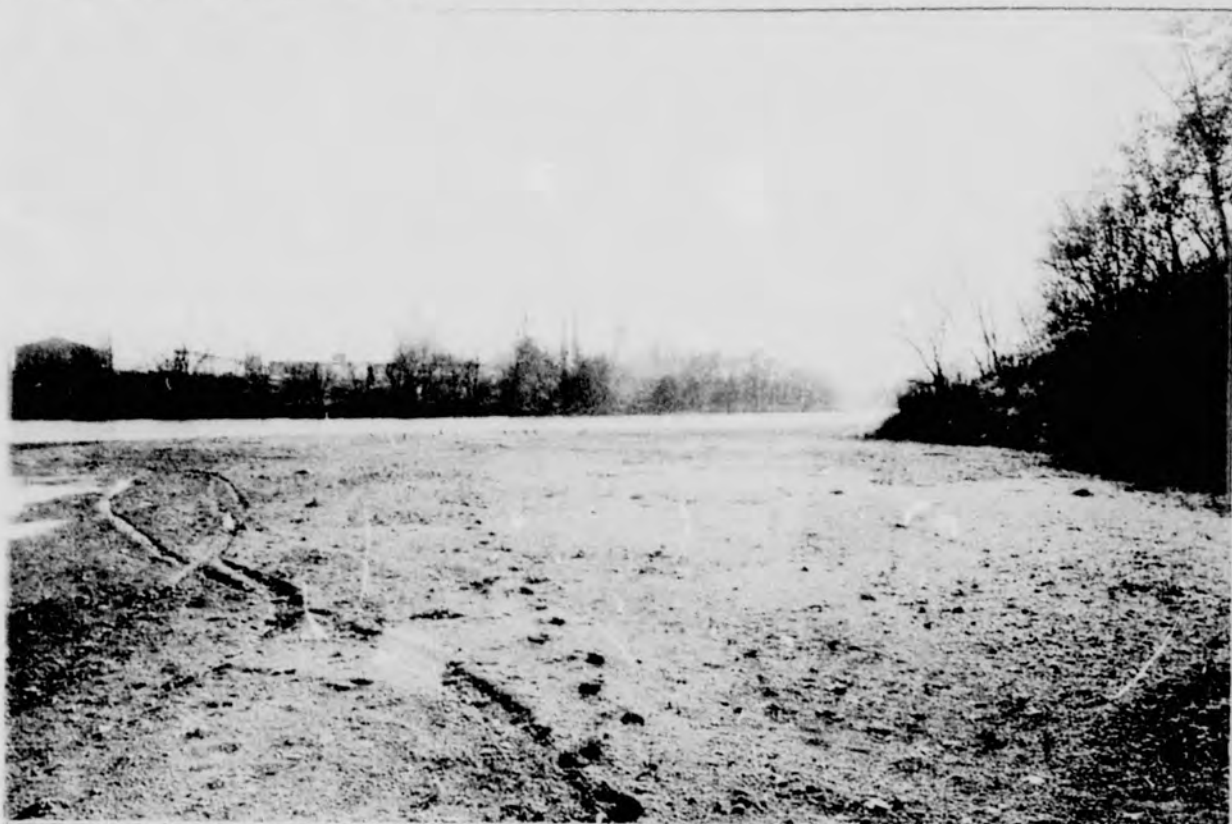
Photo D - View in the vicinity of the end of the bridge. Note the overhead power line to the right of the picture. Overhead power line would have to be adjusted to provide adequate vertical clearance for the track over the levee
